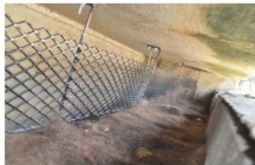
Inlet Guard with hair mat inside a storm drain
