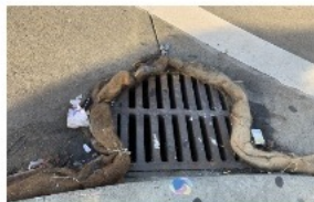
50% of oil in our waterways enters via storm drains
