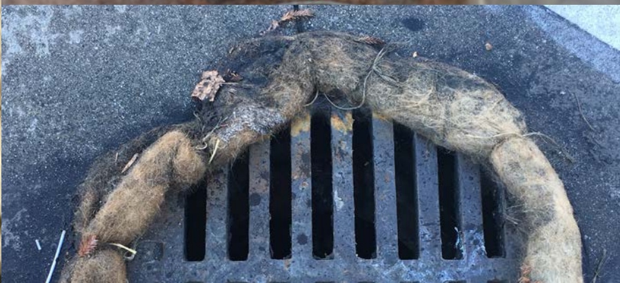
City storm drain lined with mat
